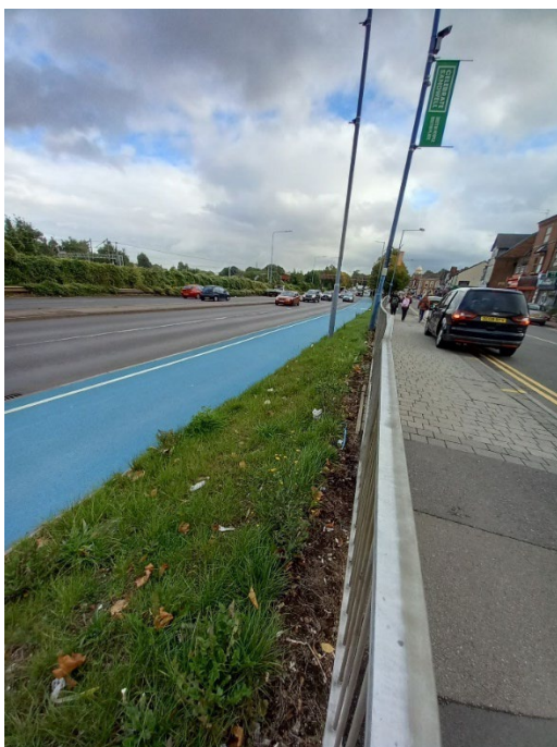
Figure 2.13 A457 Cycle Lane (phase 2 extension under construction)
