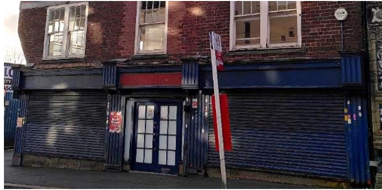
Figure 52 22-24 Lower High Street.
