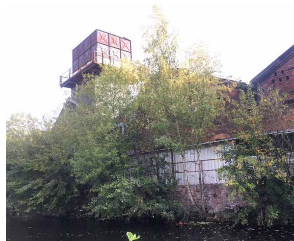
Existing water tower
