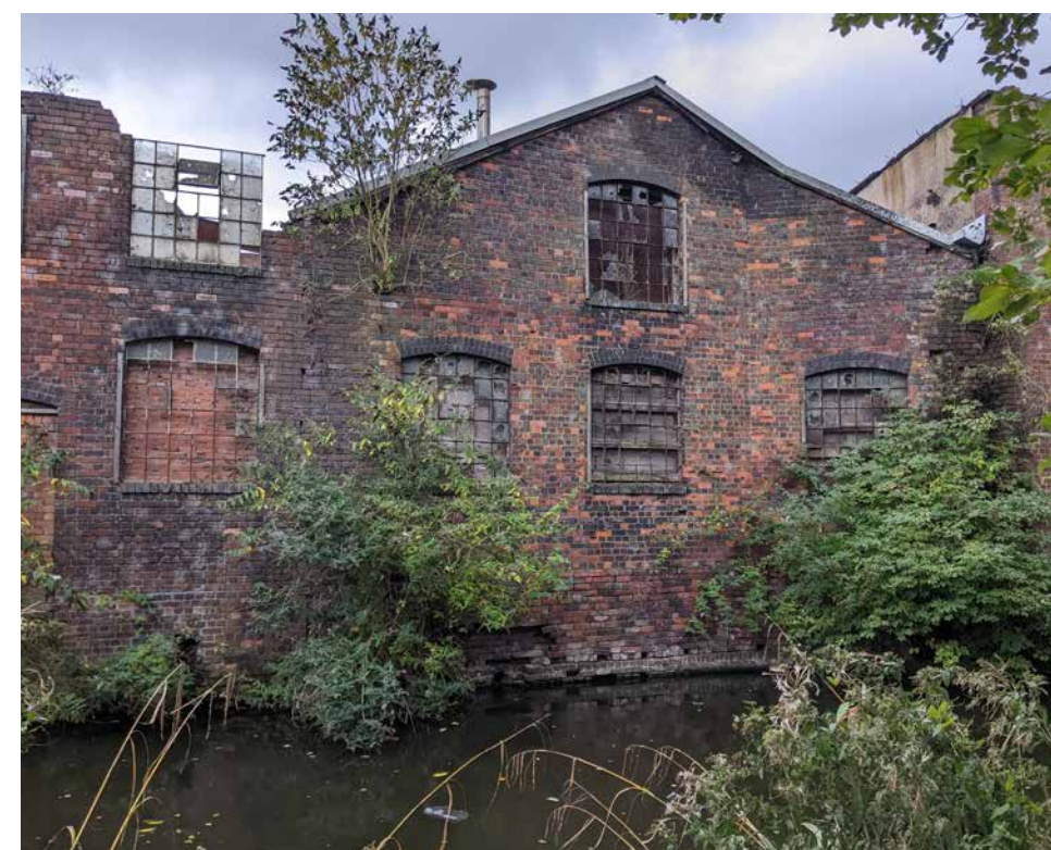
Existing warehouse elevations onto the Engine Arm
