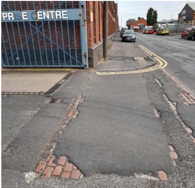
Plate 2.46 Covered pavers at the entrance to the Enterprise Centre
