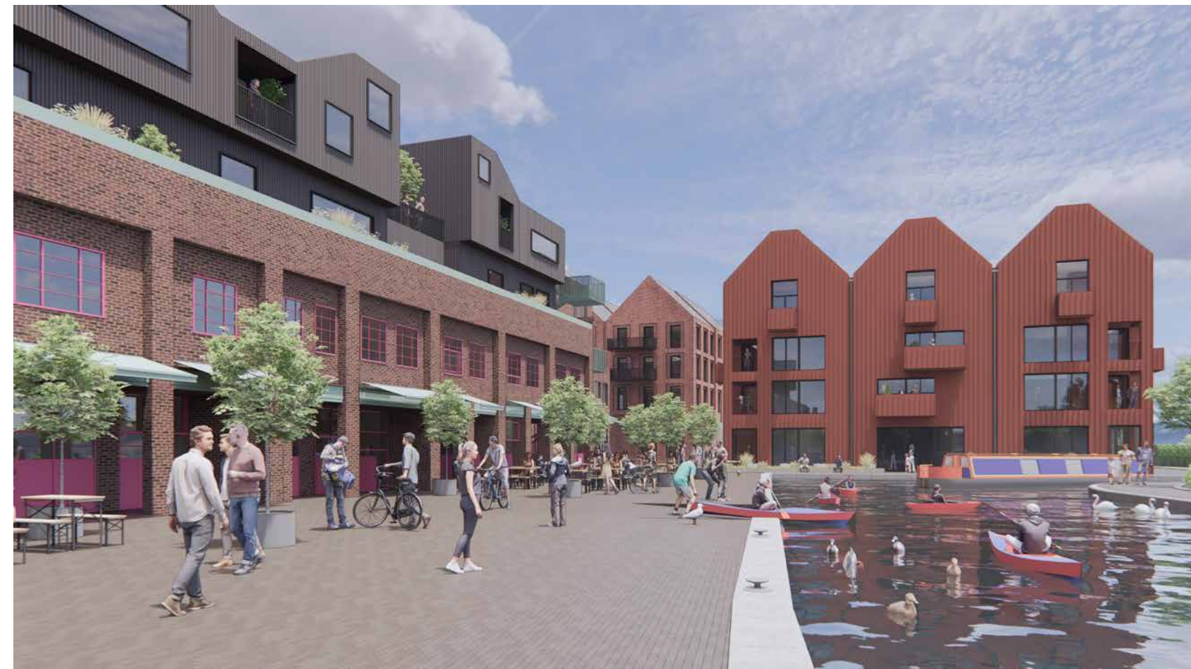
Corporation Yard – Waterside View
