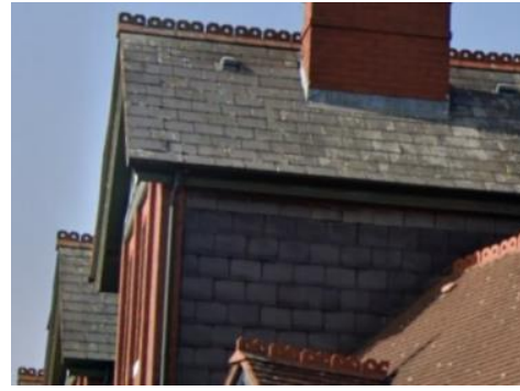
Figure 49 Decorative Ridge tiles, Upper High Street
