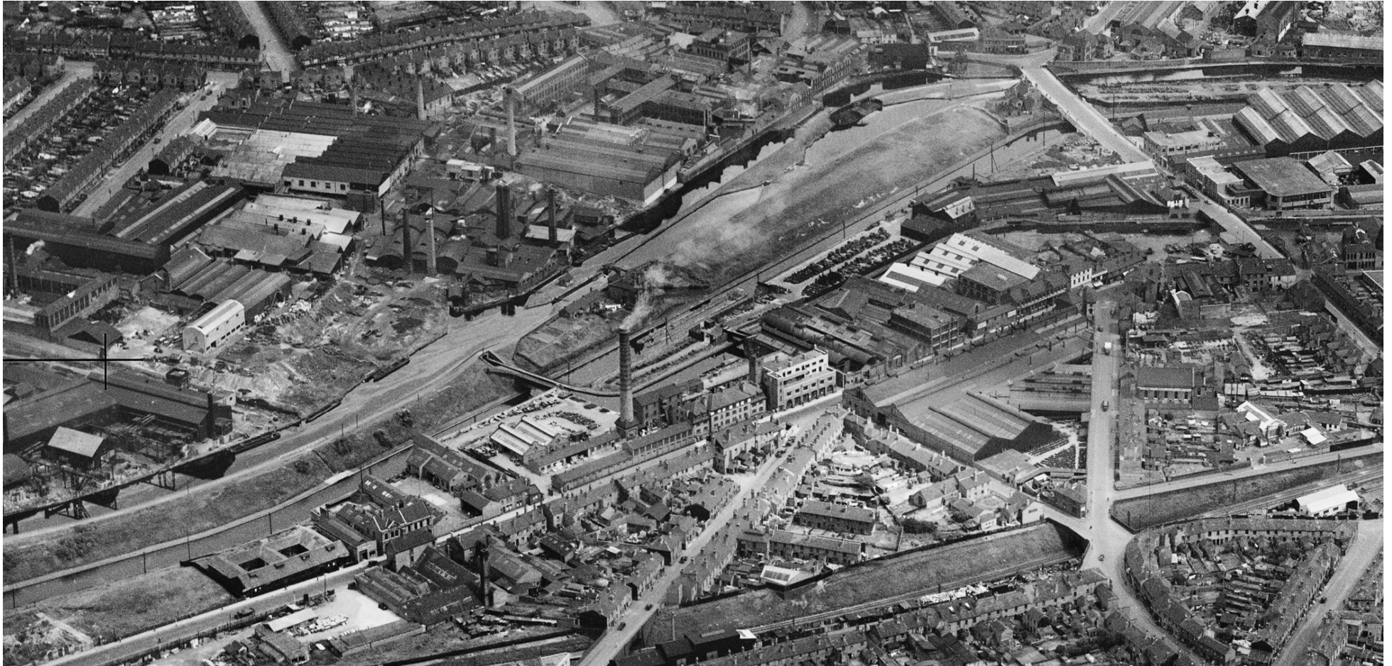
Plate 2.1 Aerial Photograph of the masterplan area 1946 © Historic England Archive. Aerofilms Collection
