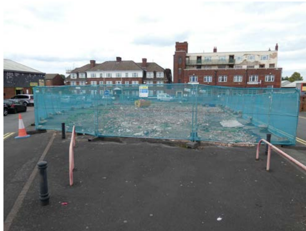
Plate 2.6 Site of the Crown and Anchor, demolished 2022
