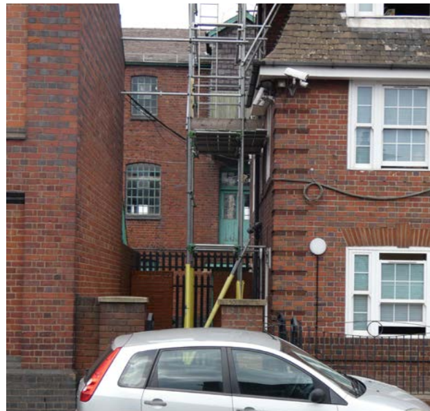
Plate 2.20 Glimpse to industrial buildings on the Enterprise Centre site
