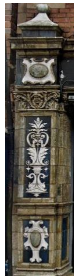
Figure 45 Pilaster, former Turks Head
