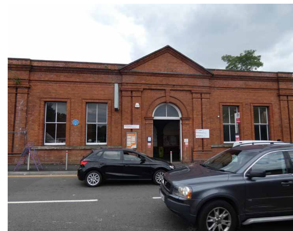
Rolfe Street station building
