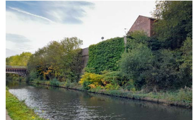
Plate 2.48 The retaining wall to the Corporation Yard along the New Main Line covered with vegetation
