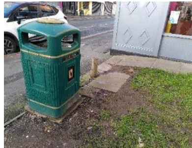
Figure 74 Degraded public realm, Lower High Street
