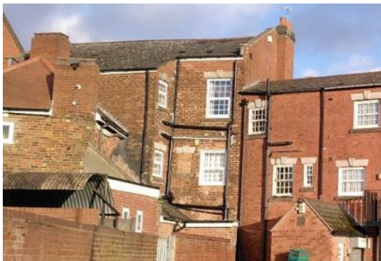
Figure 21 Rear of properties along Lower High Street
