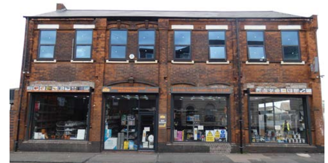
Plate 2.18 80 Rolfe Street with carriage opening
