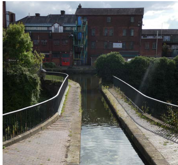
Plate 2.62 Engine Arm Aqueduct from the Old Main Line
