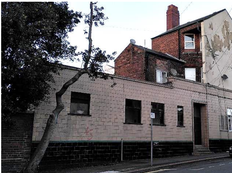
Figure 78 Former Public Conveniences, The Shambles
