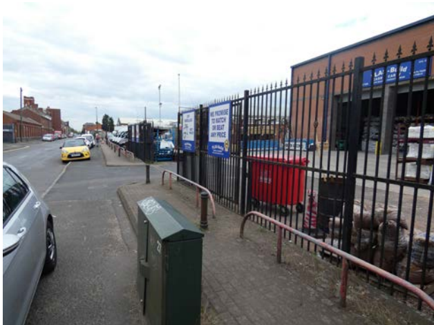
Plate 2.5 Built form is set well back from Rolfe Street behind modern boundary fencing
