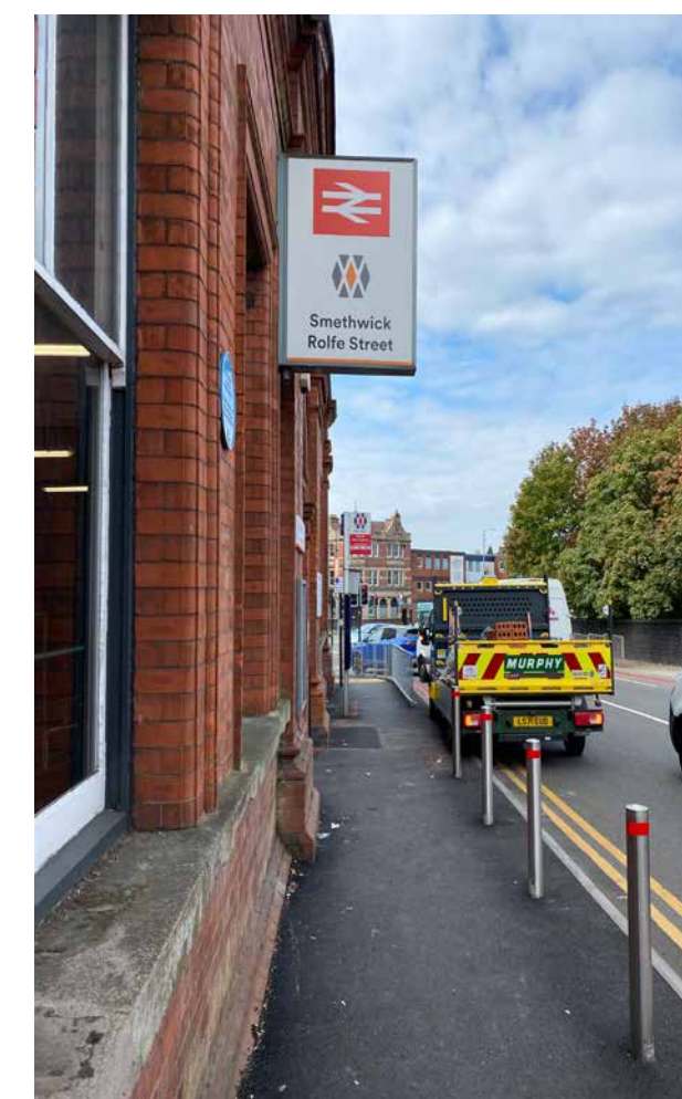
Challenging pedestrian environment at Rolfe Street Station
