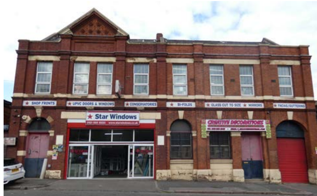
Plate 2.12 Former Post Office
