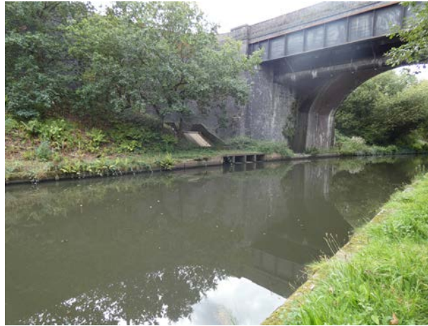
Plate 2.52 Brasshouse Lane Bridge
