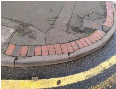
Figure 73 Paving Russell Street
