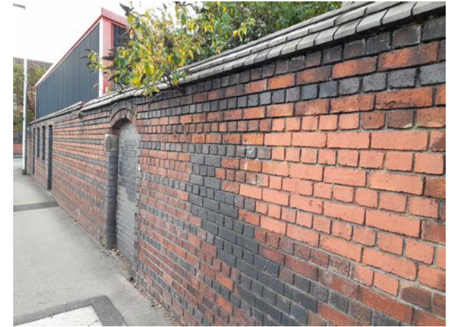
Plate 2.8 Wall to the site of the Smethwick Engine
