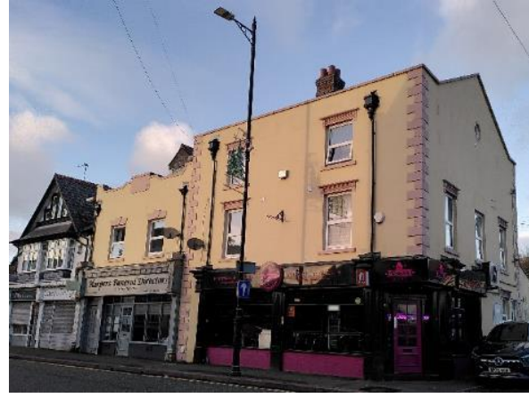
Figure 84 Buildings and shopfronts, Upper High Street
