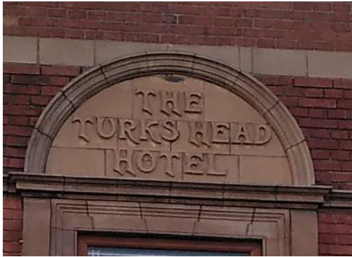
Figure 53 (Former) Turks Head Hotel 25-26 Lower High Street
