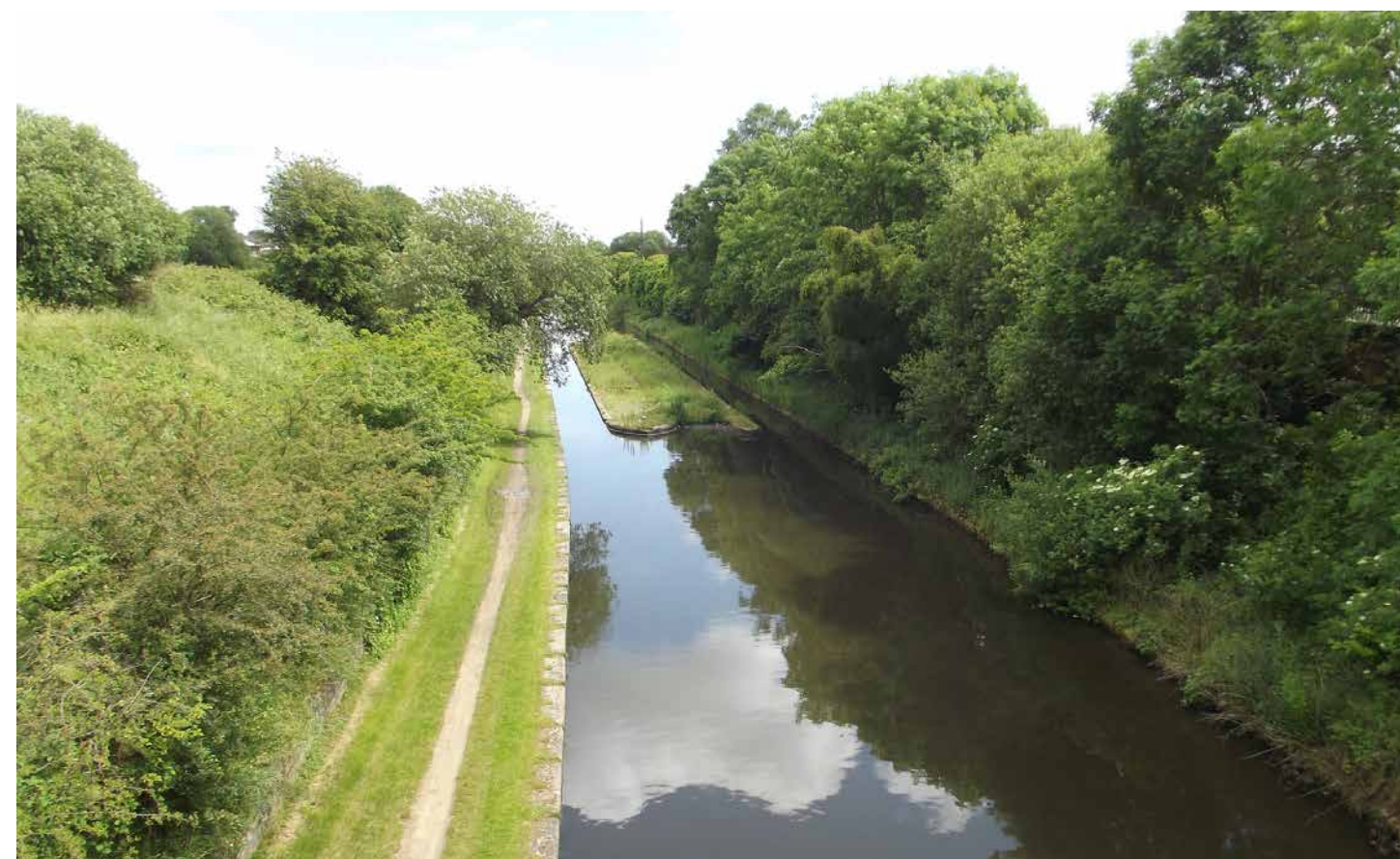
The New Main Line from the Engine Arm Aqueduct
