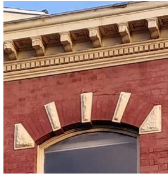
Figure 48 55 Lower High Street
