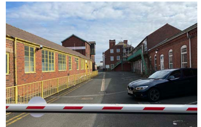
Plate 2.40 Long ranges at the Enterprise Centre site
