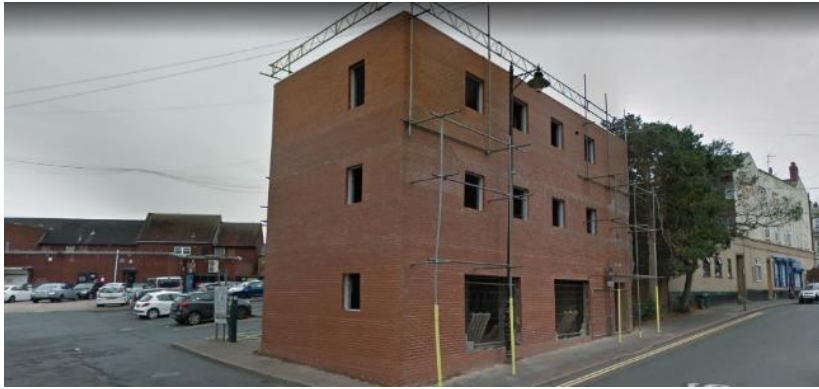
Figure 79 Unfinished building, The Shambles. Google Streetview.
