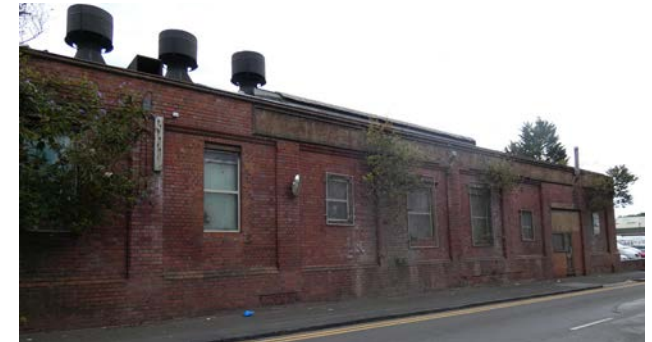
Plate 2.17 Former Drop Forge Works
