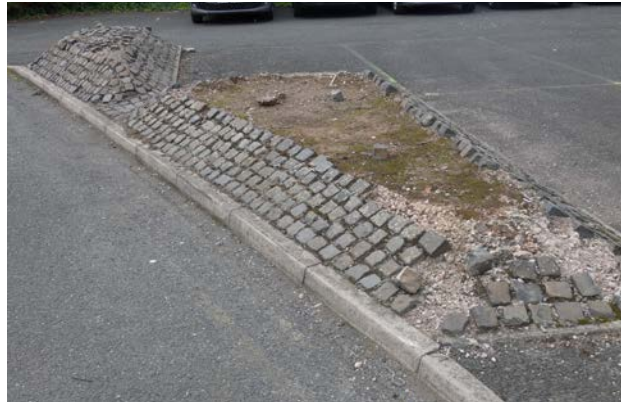
Plate 2.47 Setts close to the Engine Arm at the Enterprise Centre site
