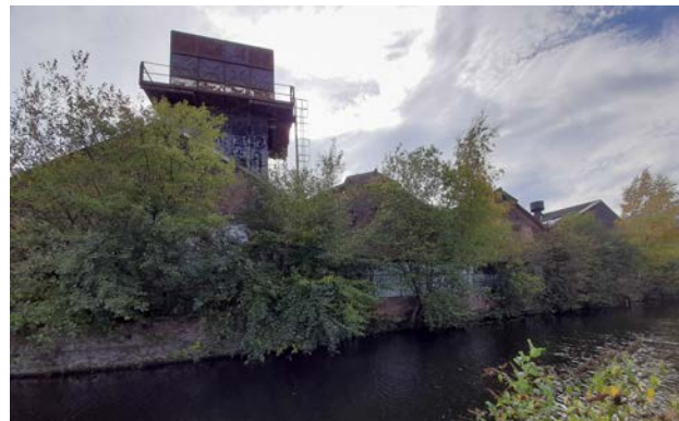
Plate 2.35 Industrial buildings fronting the Engine Arm, with prominent water tower
