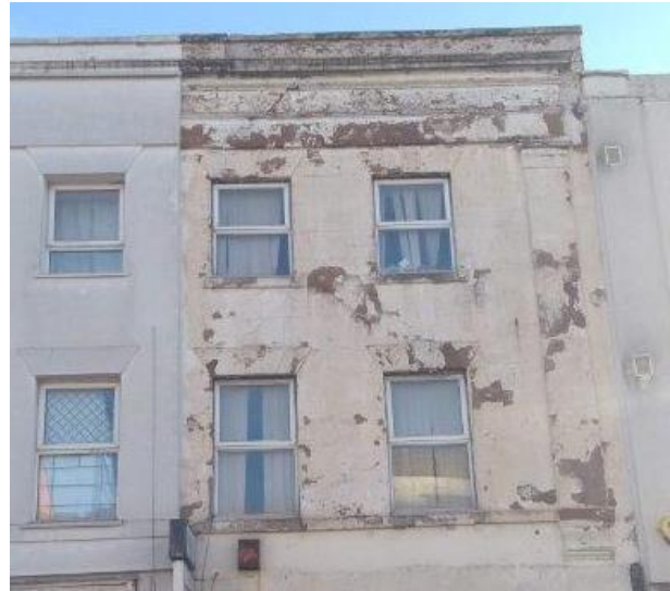
Figure 42 43 Lower High Street
