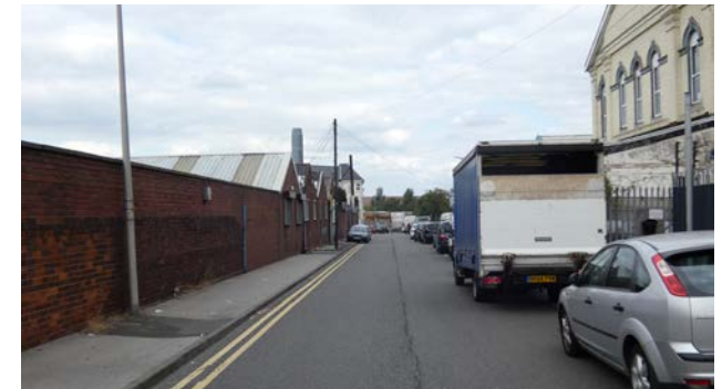
Plate 2.27 New Street with the gables of the Drop Forge Works (left) and Wesleyan Chapel (right)
