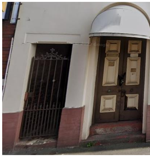
Figure 39 55 Lower High Street
