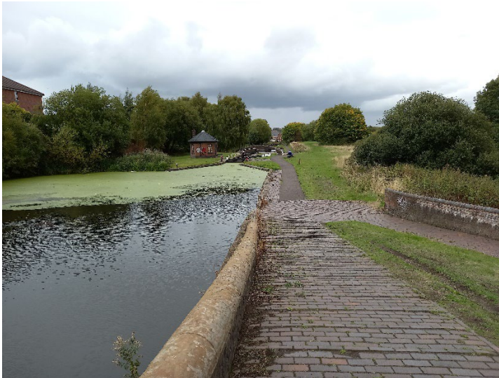
Figure 2.12 Canal side cycle provision
