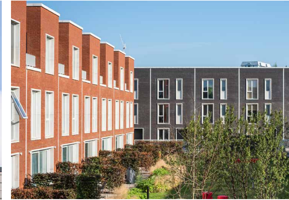
Materiality, window and metalwork detailing at Port Loop, Birmingham
