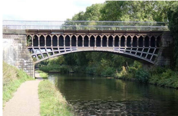
Plate 2.61 Engine Arm Aqueduct from the New Main Line
