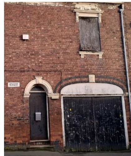
Figure 40 56 Lower High Street
