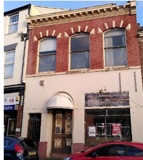
Figure 81 Poor quality signage, Lower High Street.
